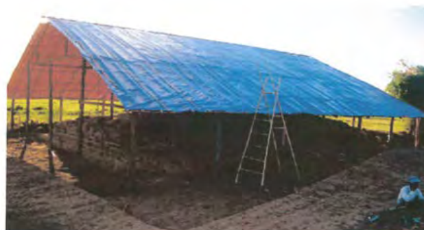
Fig. 31: Completion of temporary site shelter.
